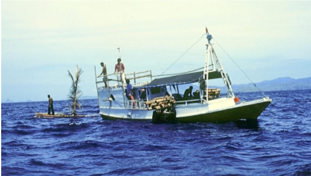
Installation of a Fish Aggregating Device, using a local boat and locally available materials. The boat is specially rigged to transport the anchors of the FAD.
