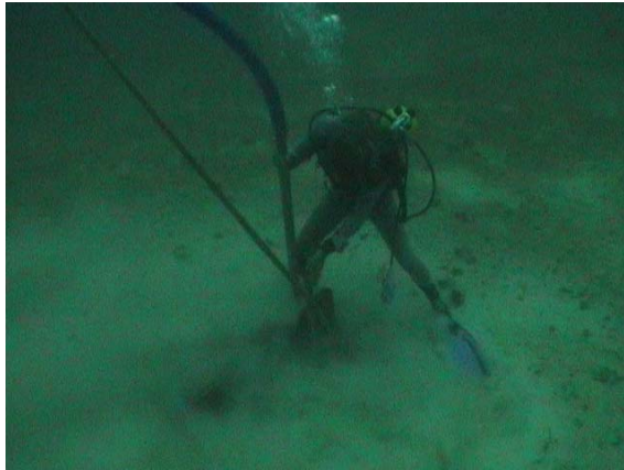
Figure 12. SCUBA diver using a water jet to sink an anchor of one of the moorings into the sand.
