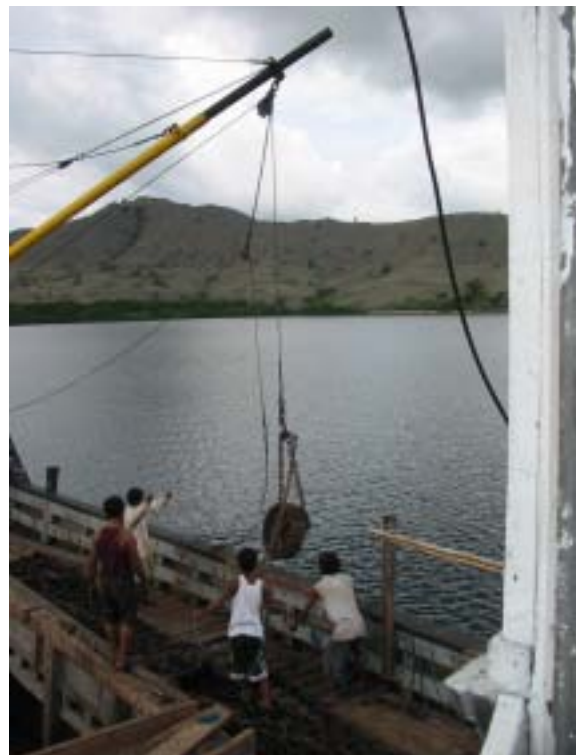
Figure 11. Ground tackle for 'Small Boat' moorings being deployed by the MV 'Duta Daerah'.
